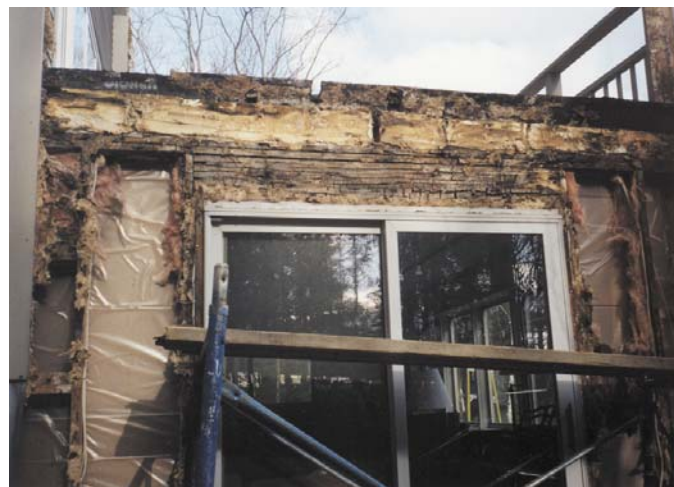
Photograph 5: Failure on Steroids —Note the plastic vapor barrier “accelerant” in this Vancouver, Canada building.
