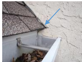
No Kickout Diverter
