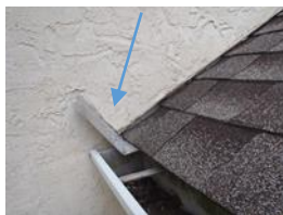
Kickout Diverter
