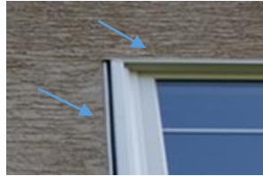
Head Flashing & Soft Joint
