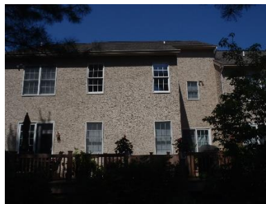
No expansion/control joints
