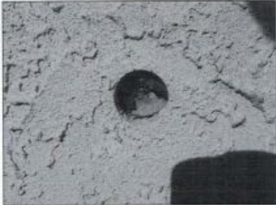
3.0 Item 1(Picture) Core sample confirms Thermo Ply Substrate & tar paper for the WRB
