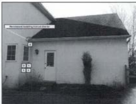
2.4 Item 2(Picture) Right rear Findings
