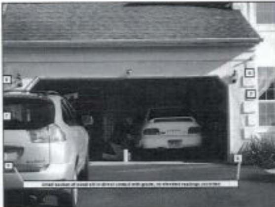
2.1 Item 1(Picture) Front left Findings
