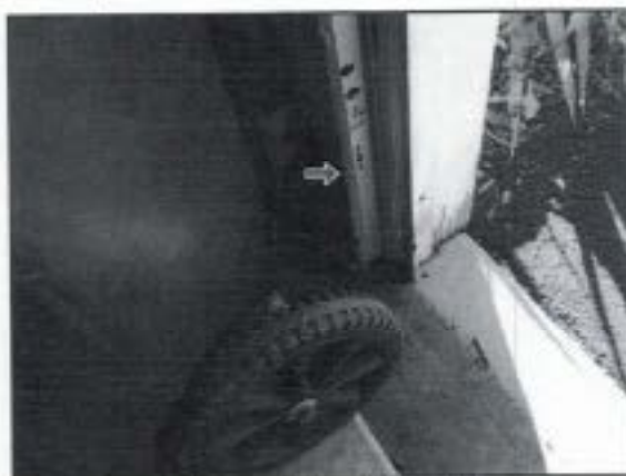
3.0 Item 7(Picture) Small sill plate at grade on left & right of garage doors
